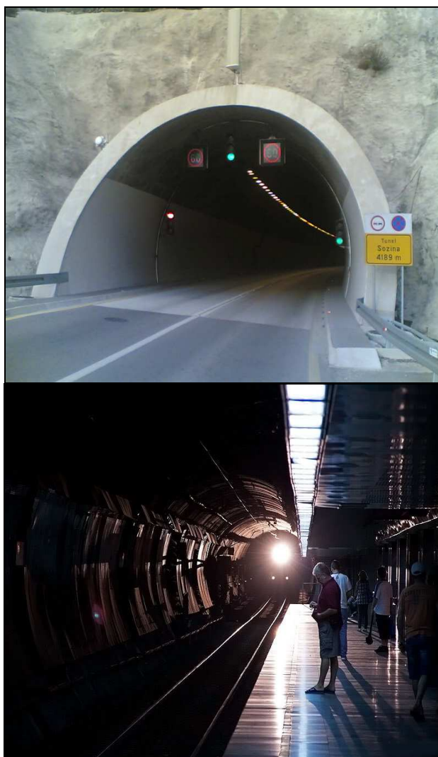
Figure 1. Tunnel Sozina in Montenegro (left) and tunnel of Belgradesubway (right) (figure source: https://www.google.rs/search?q=zeleznicki+tuneli&espv=2&biw=1280&bih=685&tbm=isch&tbo=u&source=univ&sa=X&ved=0CBoQsARqFQoTCICZt7vFwcgCFQK8GgodGNQNiw )
